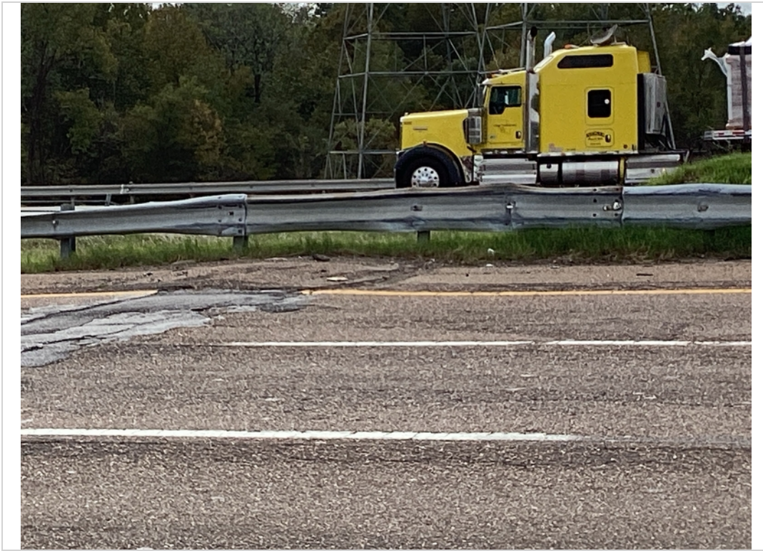
Approach 2 right transition damage
