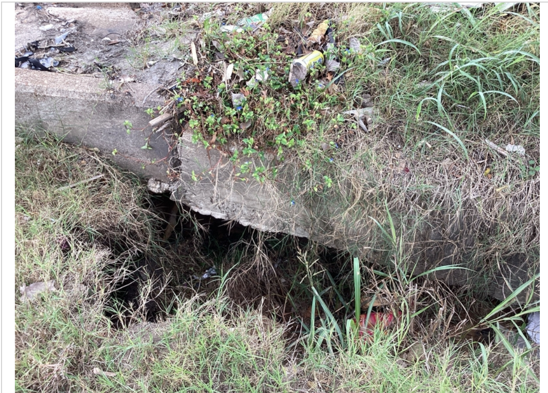
Approach 1 left embankment washing below and under drain
