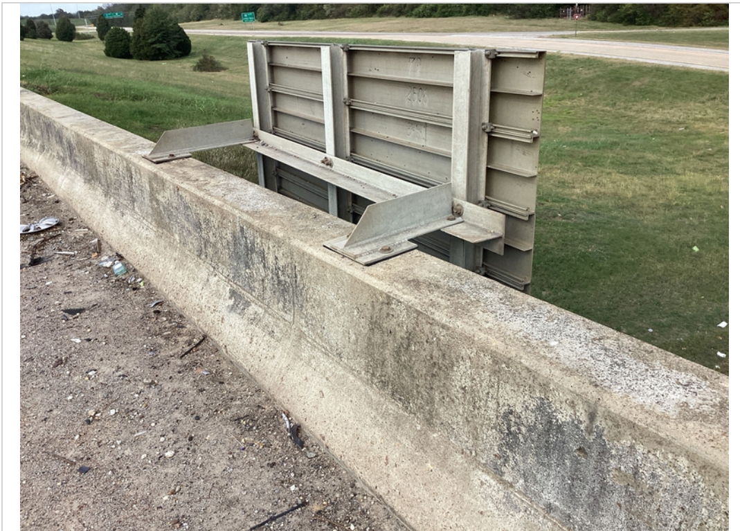
Bridge mounted sign upper connection
