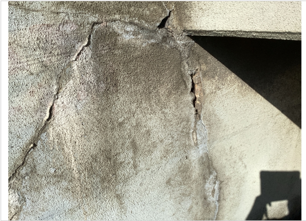
Abutment 1 spall to steel
