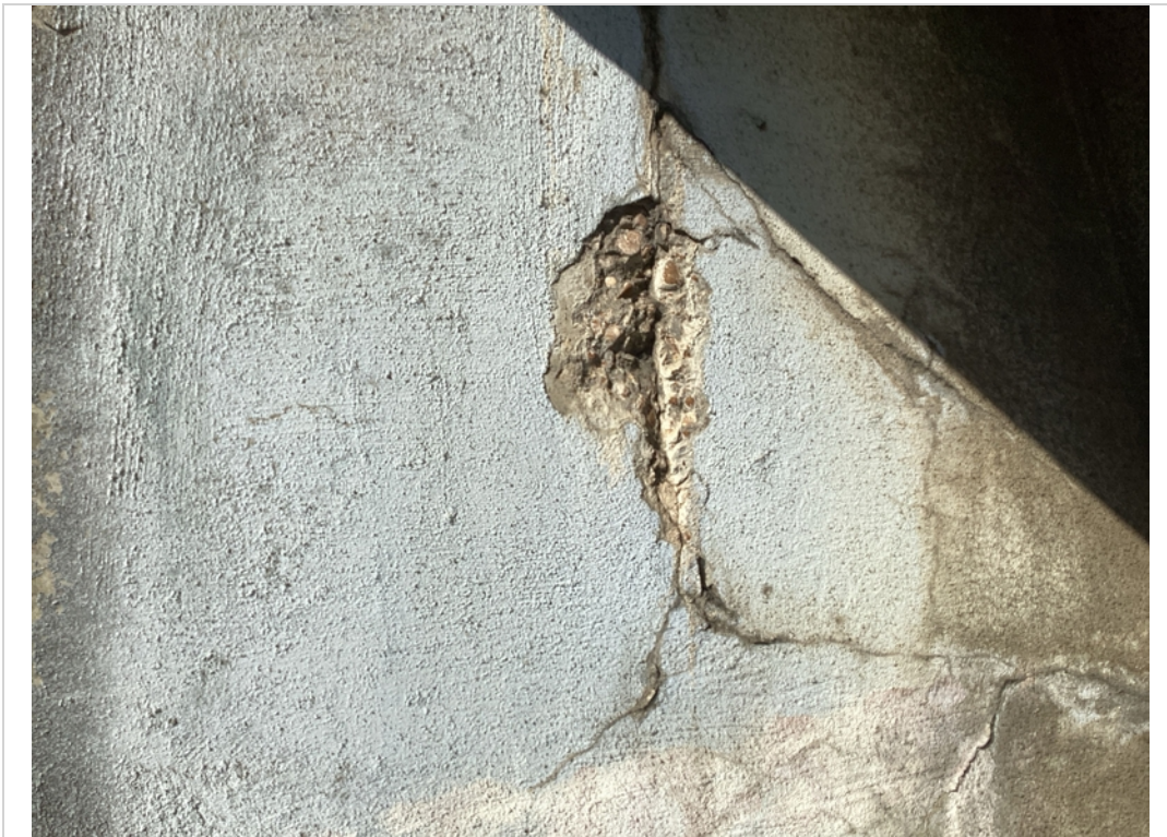
Abutment 1 spall
