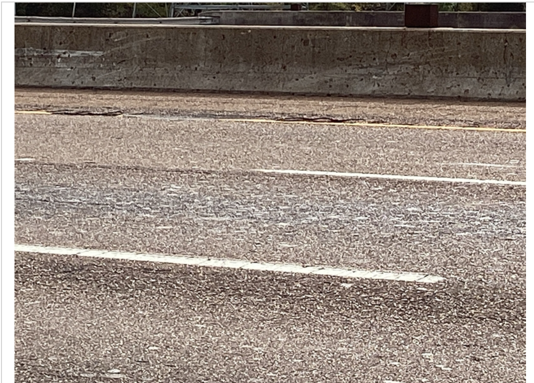
Span 1 potholes
