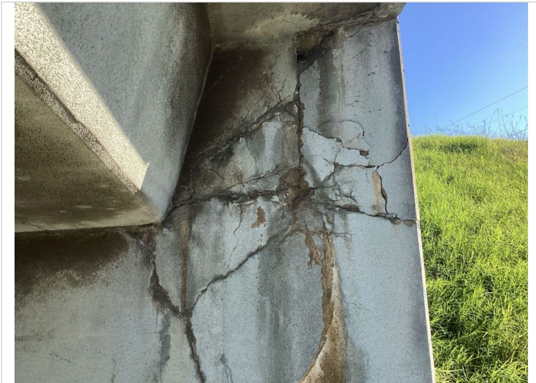
Abutment 2 , impending spall , spalling , 1/4" cracks
